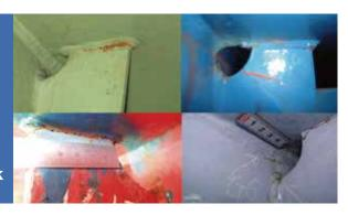
In recent years, fatigue damage cases have been reported in bridges and other structures located on heavily trafficked routes. Fatigue damage in steel road bridges varies widely in damage patterns, causes, and countermeasures depending on traffic and structural conditions, welding quality, and other factors. Josei has earned high praise for offering comprehensive proposals covering investigation, diagnosis, and countermeasure planning for these cases.
